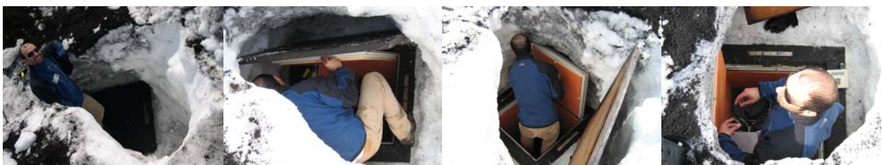
Fig. 3 – Maintenance of the BVD station during the 2006 winter.
