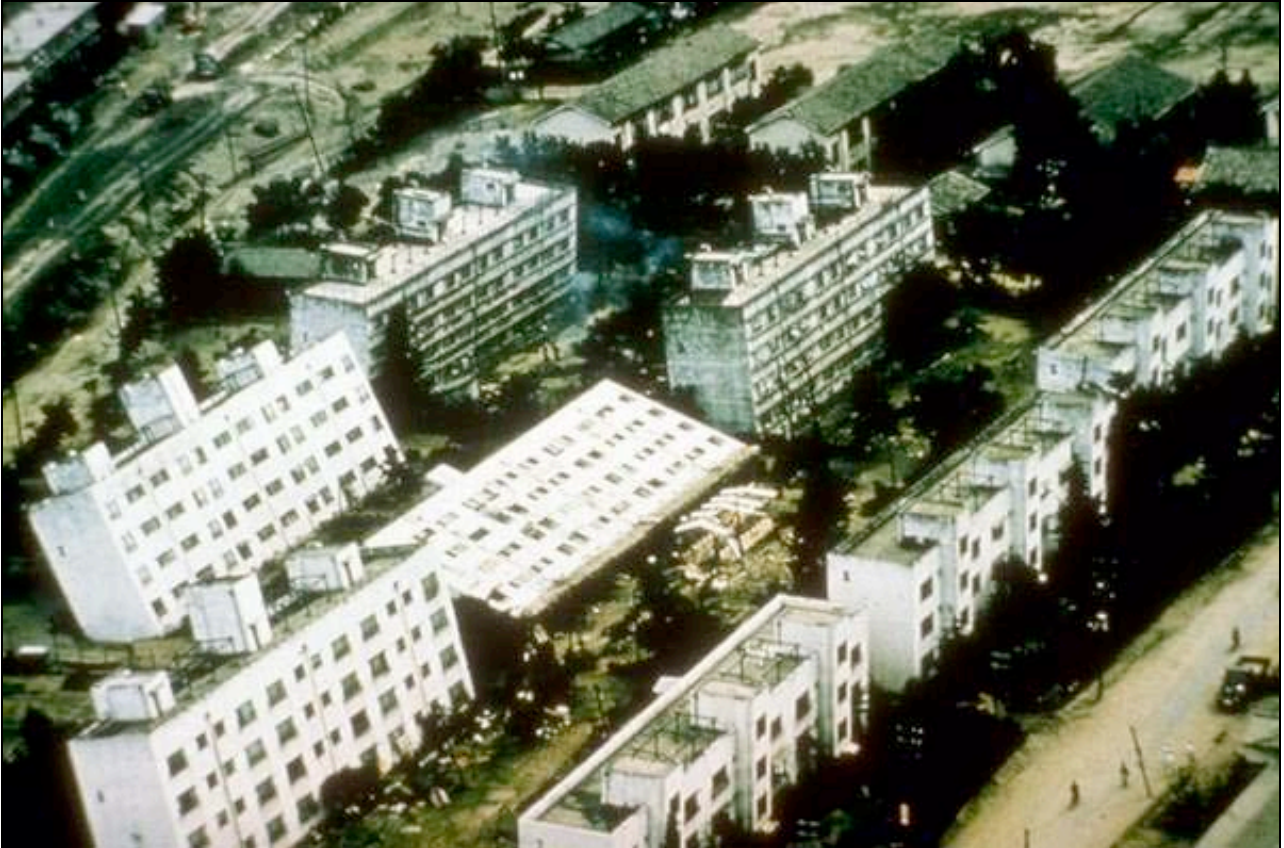
Figure 1. Aerial view of leaning apartment houses in Niigata produced by soil liquefaction. Most of the damage was caused by cracking and unequal settlement of the ground such as is shown here. About 1/3 of the city subsided by as much as 2 meters as a result of sand compaction [from: http://earthquake.usgs.gov/regional/world/events/1964_06_16.php ].
