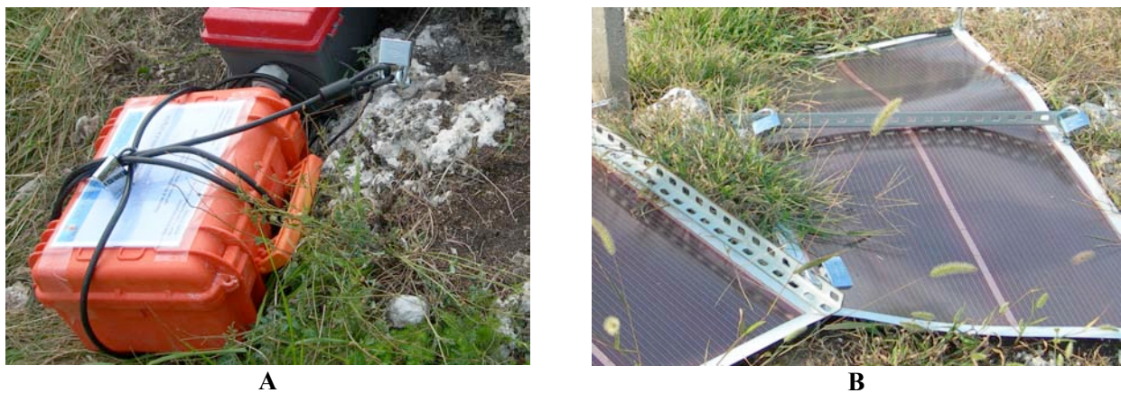
Figure 14. A: the plastic case containing the receiver secured with steel cables and steel padlocks to a metal ring fixed with epoxy in the rock outcrop (or in the concrete); B: solar panels secured by preventing the bolt steel with eyelet that to be unscrewed.
