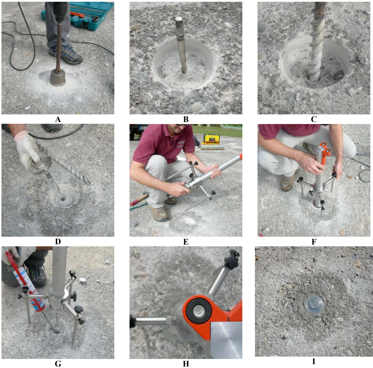
Figure 10. Realization phases of a MAX-MOUNT geodetic marker at site MT02.
