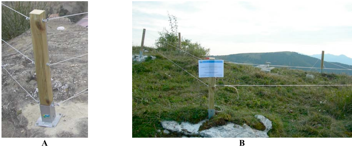
Figure 15. A: a wooden mobile pole stuck in the metal base and B: example of a light mobile fence, made by connecting wooden poles by means of steel cables.
